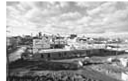
Phase One Construction
